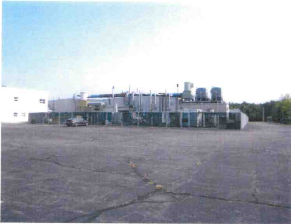
Rear of Subject Section
