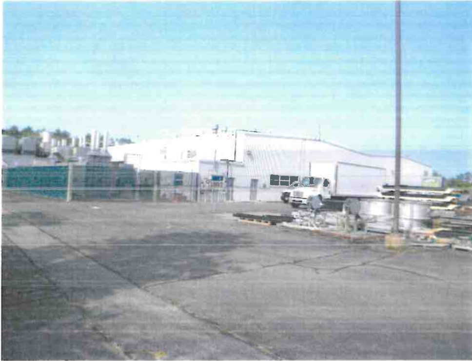
Rear of Subject Section
